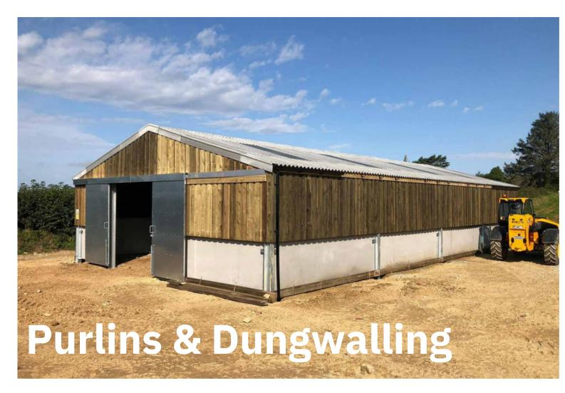
At Bond Timber we have a selection of purlins and agricultural dungwalling in stock. Timber purlins are strength graded depending on section size and load requirement.
