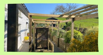
All cut ends would need to be treated with <u>Barrettine Cut End Preservative</u> also available from our shop. For fixings <u>Timberlok screws</u> were used.
