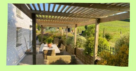
The posts are 4 x 4 planed tanalised and could be produced from either eased four corners homegrown timber or joinery unsorted redwood.
